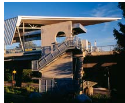
Lake City Skytrain Station, Burnaby, BC - Stantec Architecture w/ Walter Francl Arch.
